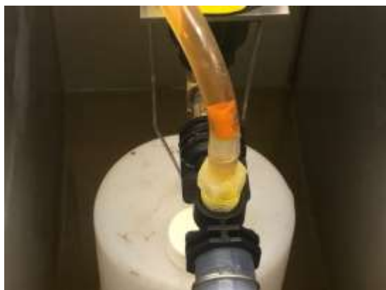
Culprit tip popped out of the barb and sitting in the tube.
