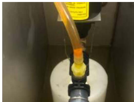
Correctly seated tip pushed home in the barb.
